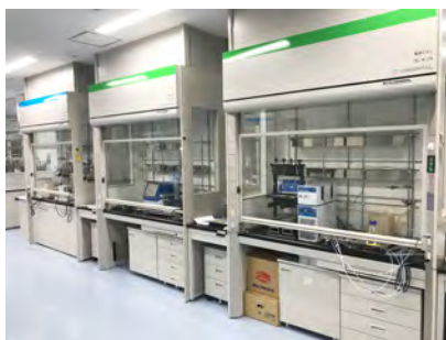
Low air volume (push/pull type), ultrahigh speed variable air volume (VAV) local ventilation device (Minase Research Institute)
