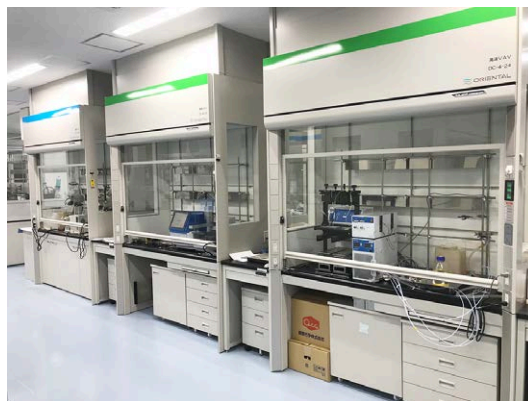
Low air volume (push/pull type), ultrahigh speed variable air volume (VAV) local ventilation device (Minase Research Institute)
