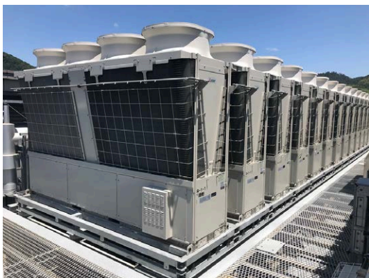
Module-type heat pump chiller (Minase Research Institute)
